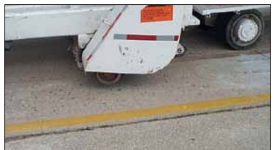
Diamond grinding of pavement lane.
