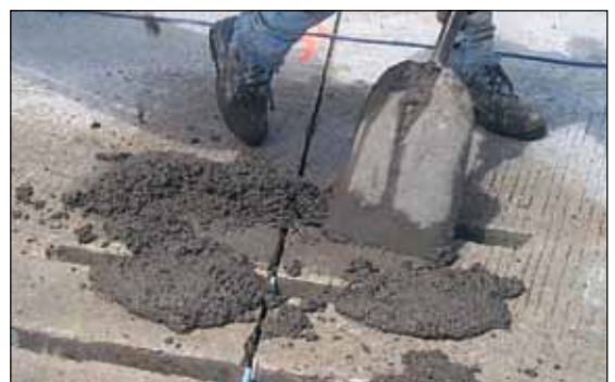
Backfilling the slots with DB Retrofit Mortar.
