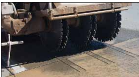
Cutting the slots (sawing).
