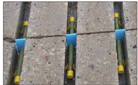
Placing the dowel bars, caps, chairs and joint filler.
